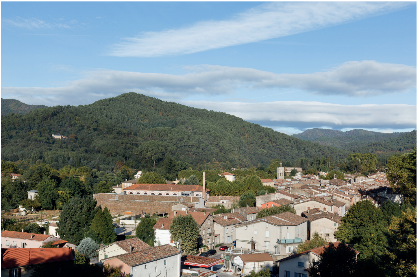
Vue lointaine aujourd'hui / View of the new building from a distance
